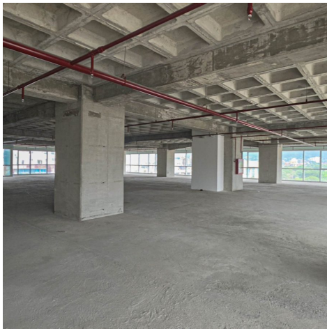
Open floor plate, 14th floor
